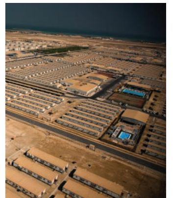
PEARL GTL, QATAR
