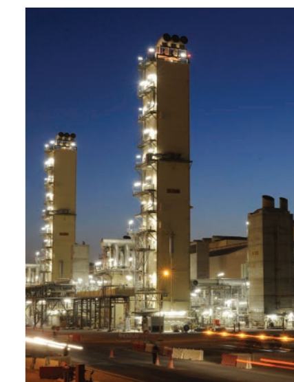
PEARL GTL, QATAR
