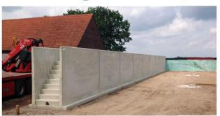
ARK Agriculture's vertical walled silage clamp system is based on a range of vertical L, T and U-shaped wall panels, specifically designed for silage clamps and the loadings of modern machinery
