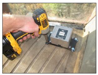
Example: Mounting in the operator's cab
