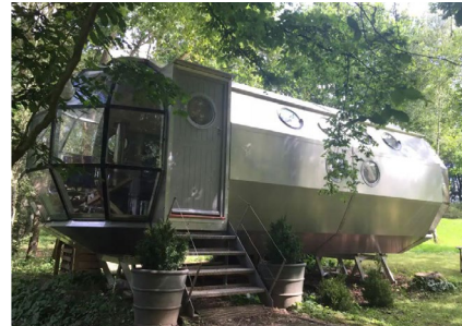
EXAMPLE 3: Prefabricated structure to be easily moved.
