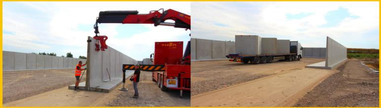
Our vertical silage clamp system is based on a range of vertical L, T and U-shaped wall panels, specifically designed to withstand the demands of modern silage storage
