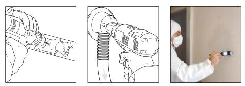
Drill through masking tape covered with paste or foam, or use a drill cowl connected to a Class H vacuum cleaner as local extraction. Seal drilled edges with sealant
